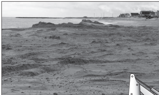
75,000 yd 3 of sand was added to storm-ravaged Town Beach, helping to rebuild public bathing areas and fortify the coast.
